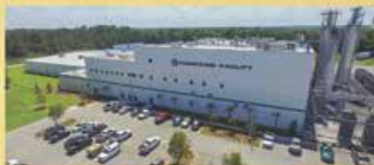
Orangburg, SC Compound Facility
